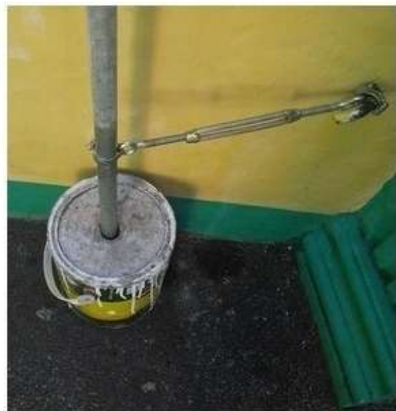
Using empty paint tin filled with cement at the base of the mast.
