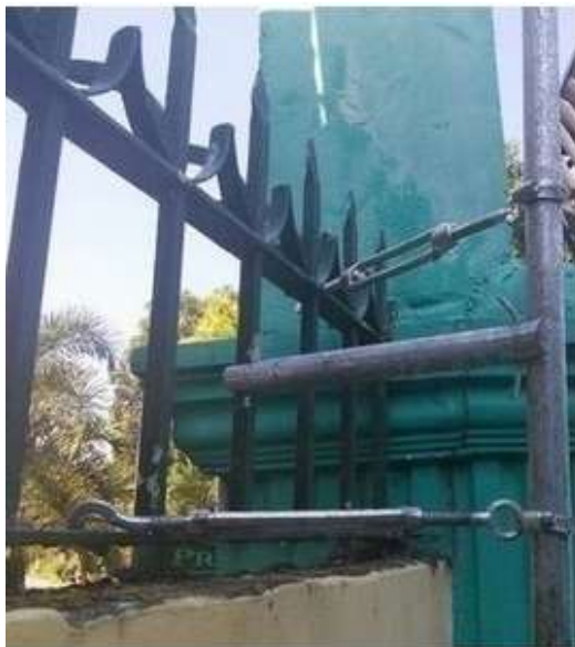
Distance piece used to secure the mast to the wall railing.
